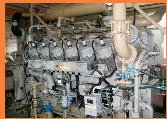
The emPact Emission Control Upgrade installed in the field at WBI Energy's Baker Booster Station in Montana.
