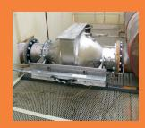
INNIO installed emPact on one of WBI Energy's Waukesha L7044GSI engines at the Baker Booster station in Montana. Performance has exceeded expectations. Seven weeks after emPact was operational, it was still maintaining emissions below 0.10 g/bhp-hr for both NOx and CO-without manual adjustment-even as site conditions changed.
